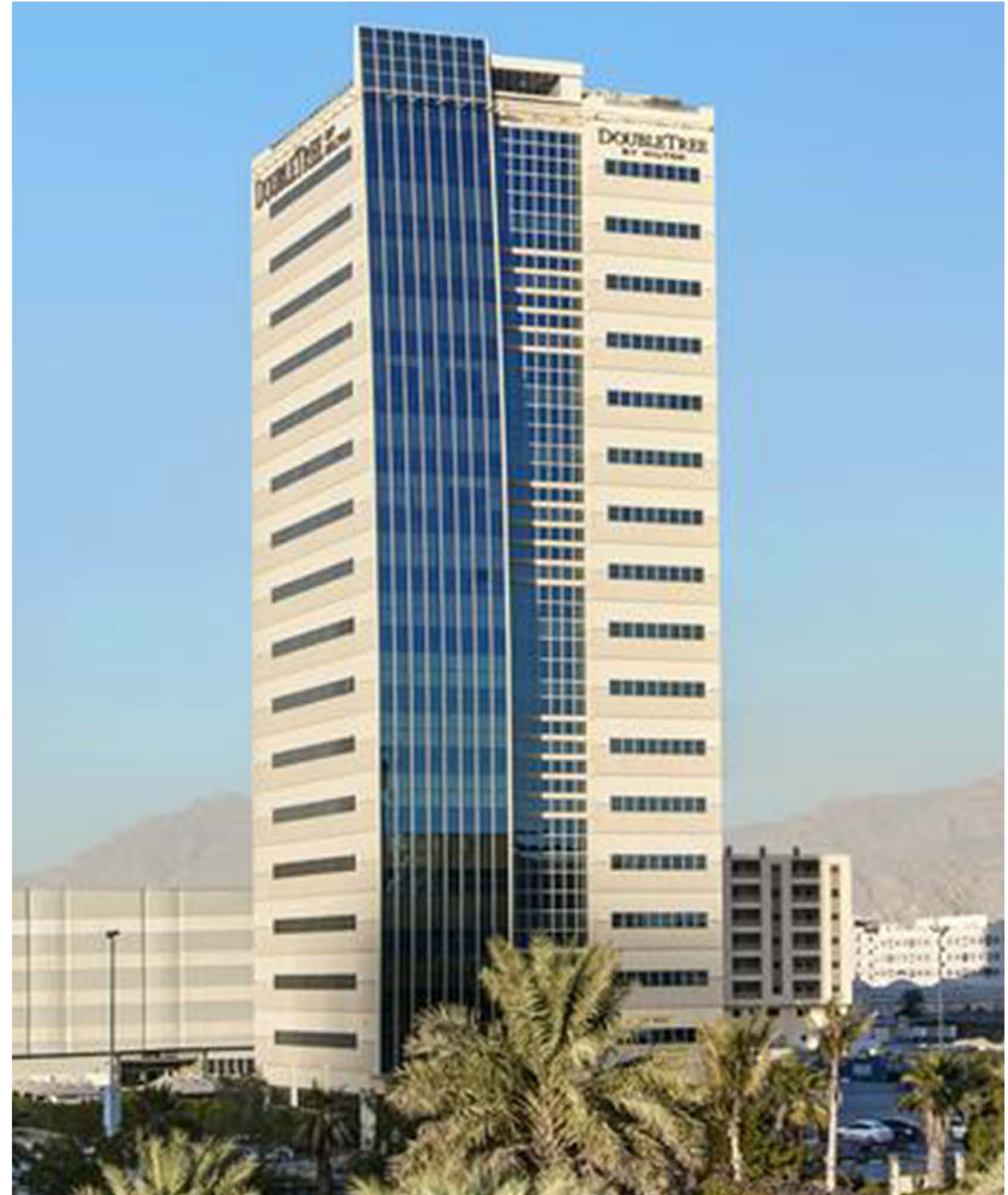
Project : Double Tree by Hilton Purpose : Hotel Apartments Location : AL Nakheel
