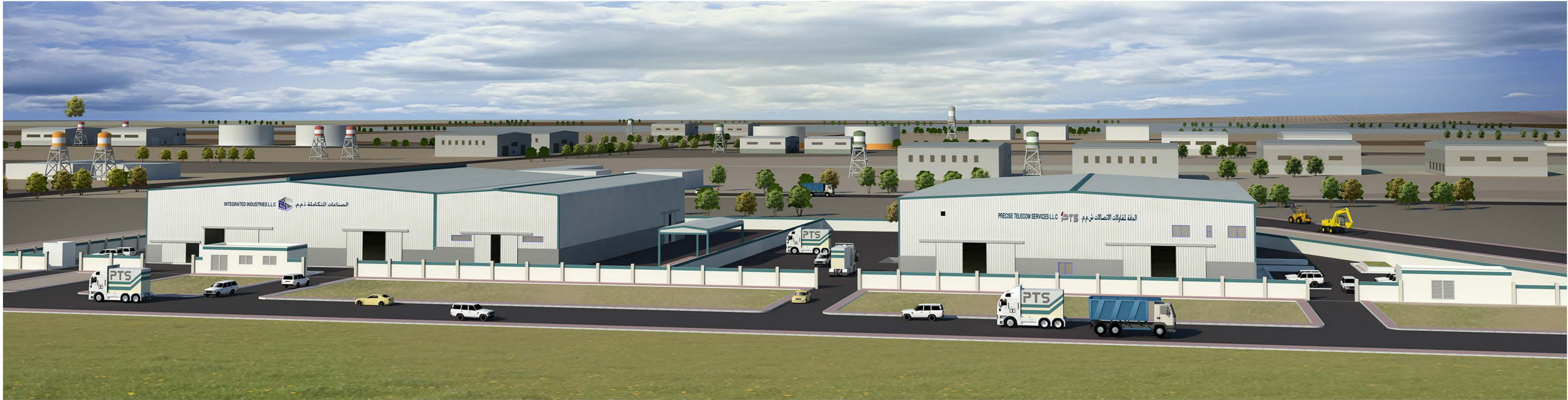
Project : Integrated Industries L.L.C and Precise Telecom Services L.L.C Location : Al Jazeera
