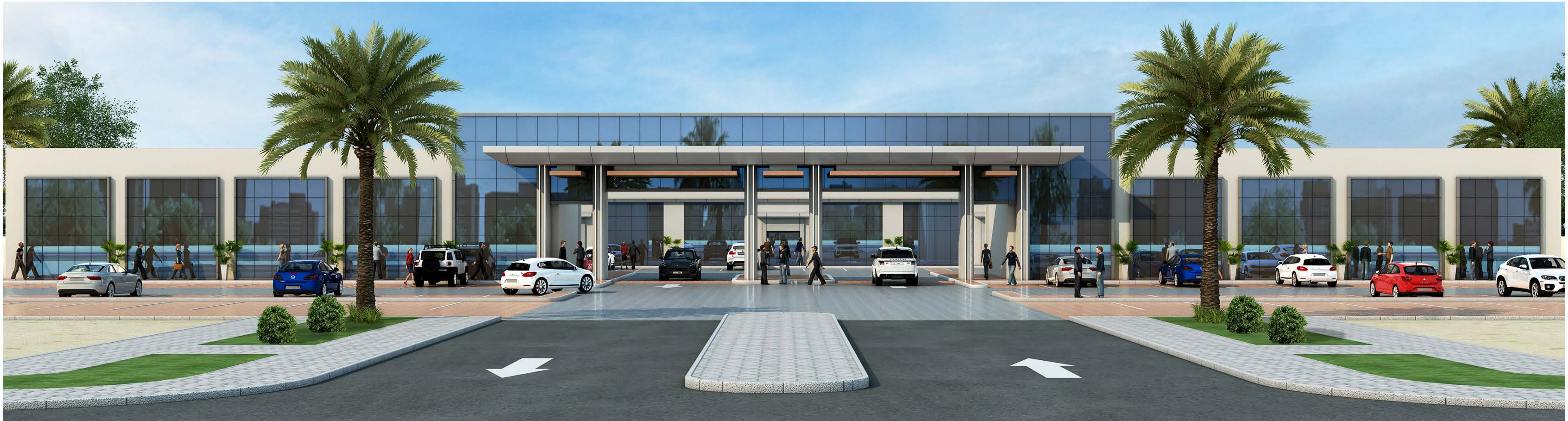
Project : Paradise Centre Purpose : Commercial Location : Al Rams
